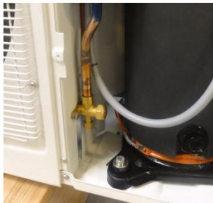
Figure 23: Liquid line service port
