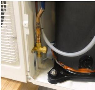
Figure 23: Liquid line service port
