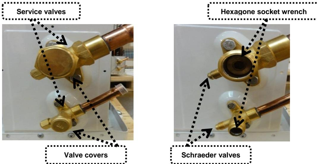
Figure 22: Service valves for refrigerant charging
