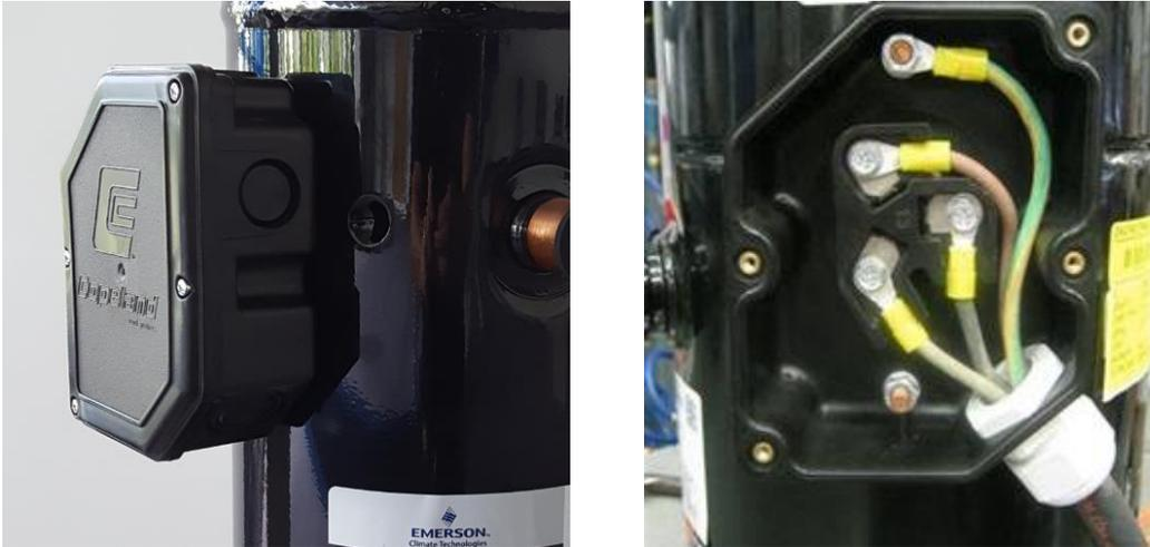
Figure 16: IP54 T-Box and correct electrical installation with cable gland
