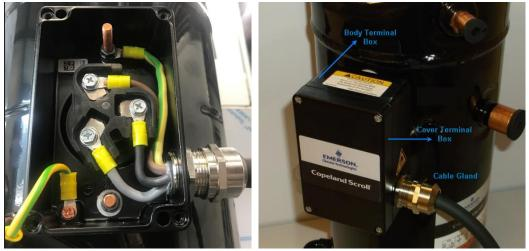
Figure 18: IP65 T-Box and correct electrical installation with cable gland
