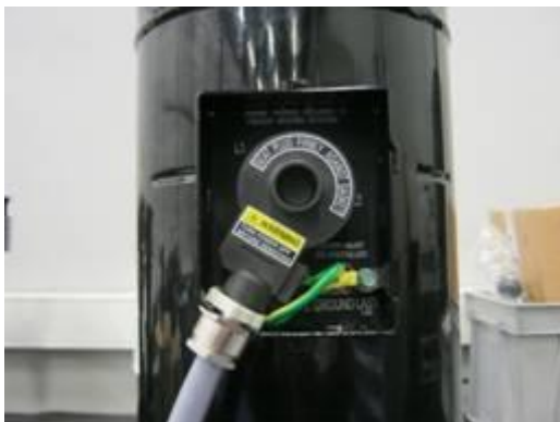
Figure 21: Terminal box IP66 and correct electrical installation with cable glands
