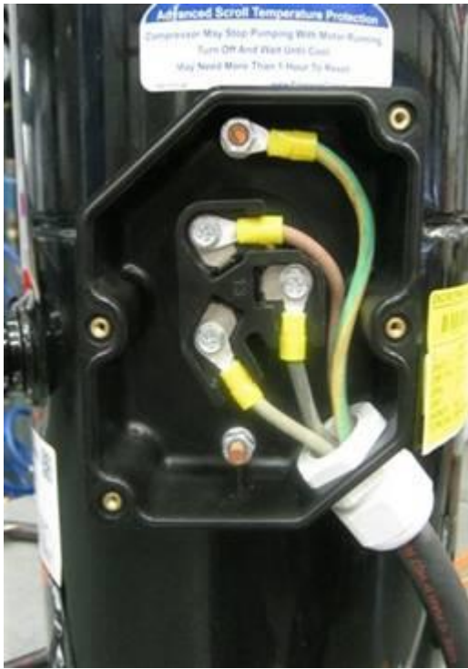
Figure 20: Terminal box IP54 and correct electrical installation with cable glands
