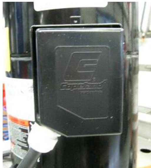
Figure 17: Correct electrical installation with cable glands for IP21 T-box (compressors ZRD61KRE to ZRD92KRE)
