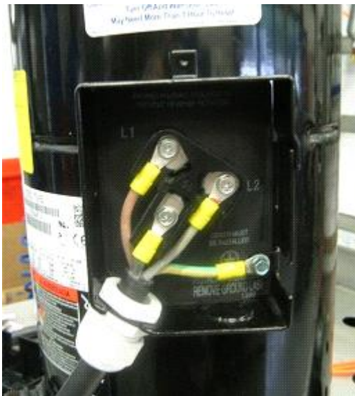
Figure 17: Correct electrical installation with cable glands for IP21 T-box (compressors ZRD61KRE to ZRD92KRE)
