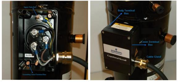
Figure 9: Terminal box and correct electrical installation
